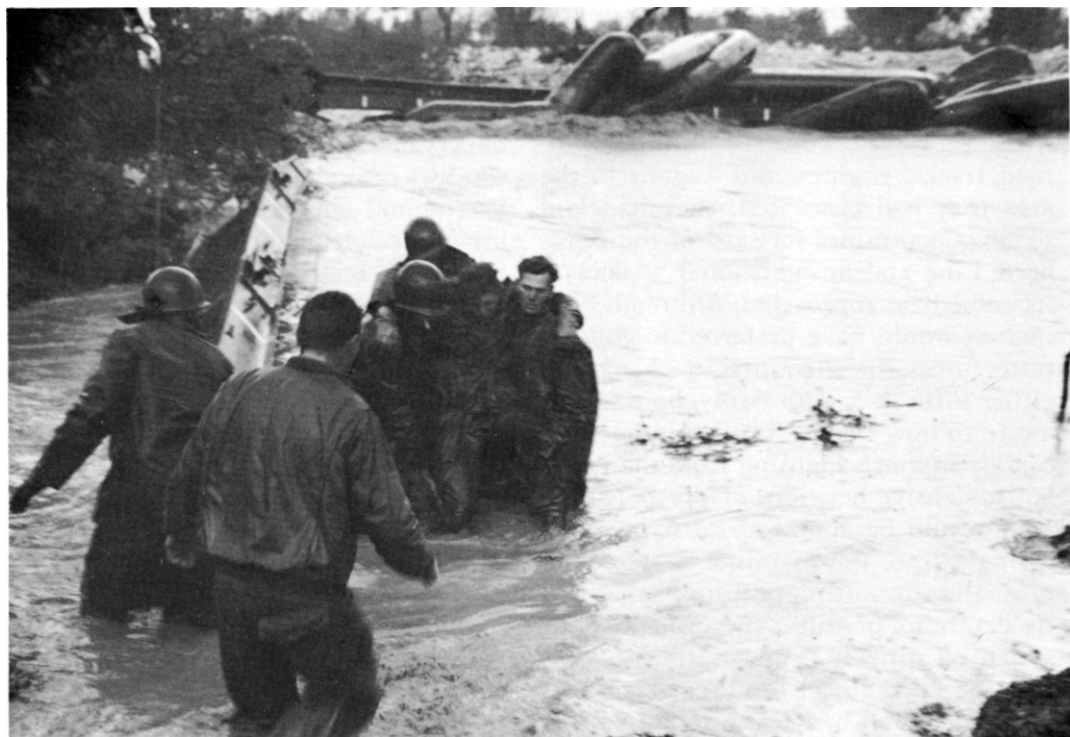
RESCUE AT THE VOLTURNO; COLLAPSED PONTON BRIDGE IN THE BACKGROUND
