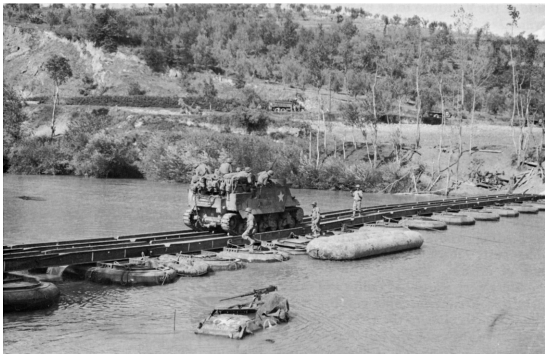
SELF-PROPELLED 105-MM. HOWITZER CROSSING THE VOLTURNO on a ponton treadway bridge.
